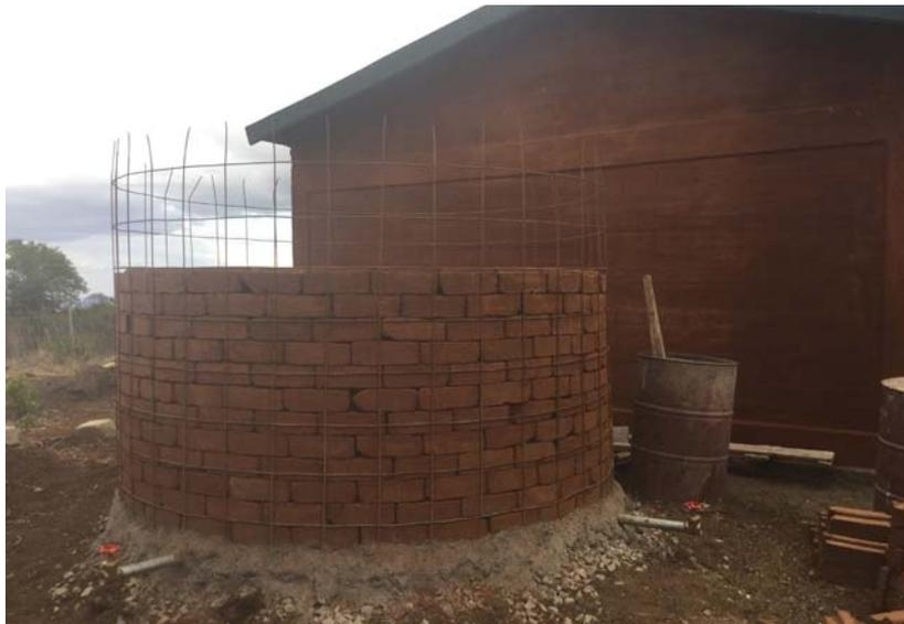
A brick water tank under construction
